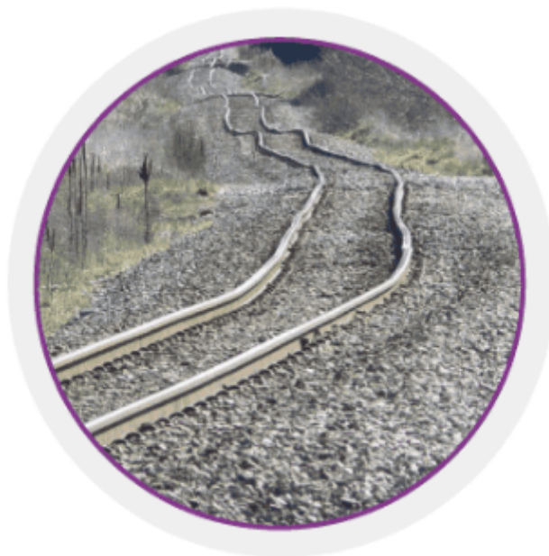
Effect of thermal expansion on railway track
